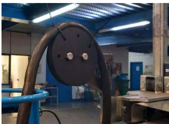
Fitting the cable on hanging bracket
